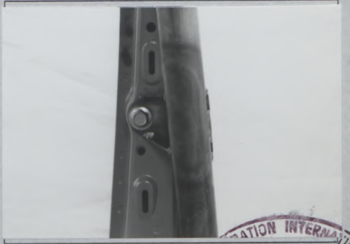
MAIN HOOP TO PILLAR
