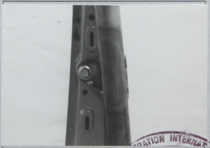
MAIN HOOP TO PILLAR
