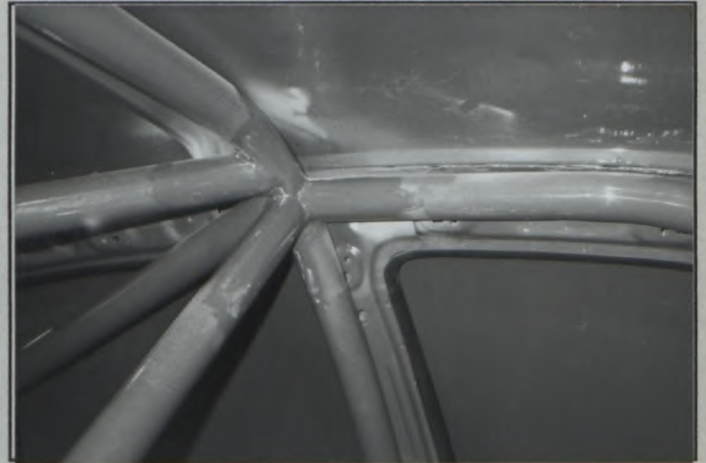
MAIN HOOP TO ROOF AND PILLAR
