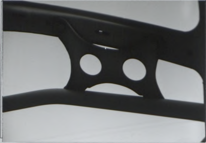
Photo No.7 Main hoop to pillar
