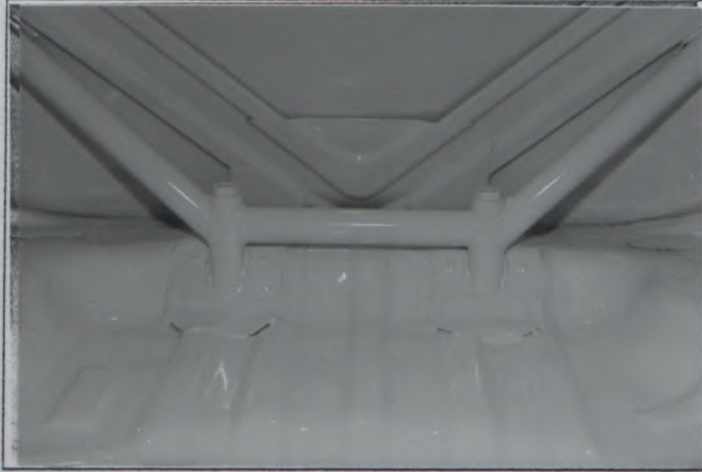
Rear framework to floor, upper
