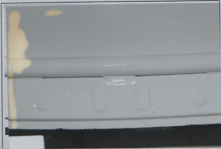
Front screen bar to roof
