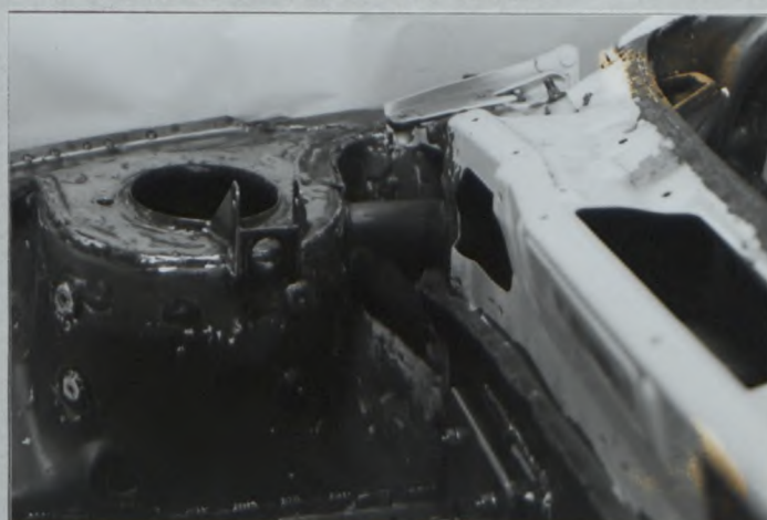
PHOTO No.12 Front framework to turret
