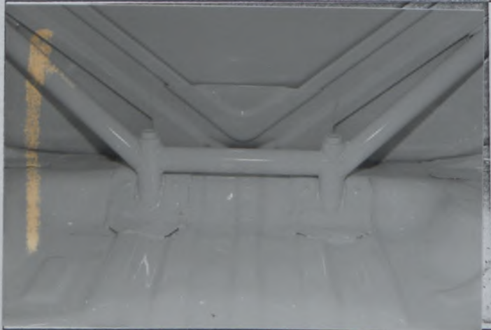
Rear framework to floor, upper
