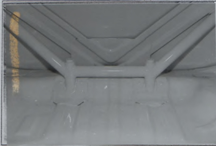
Rear framework to floor, upper
