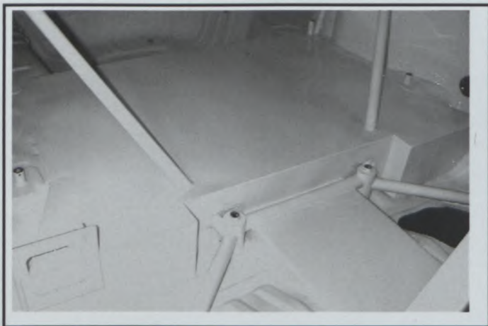
PHOTO N° 12 REAR SUPPORT TO FLOOR
