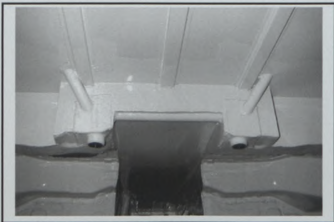
PHOTO N° 14 REAR SUPPORT TO FLOOR LOWER
