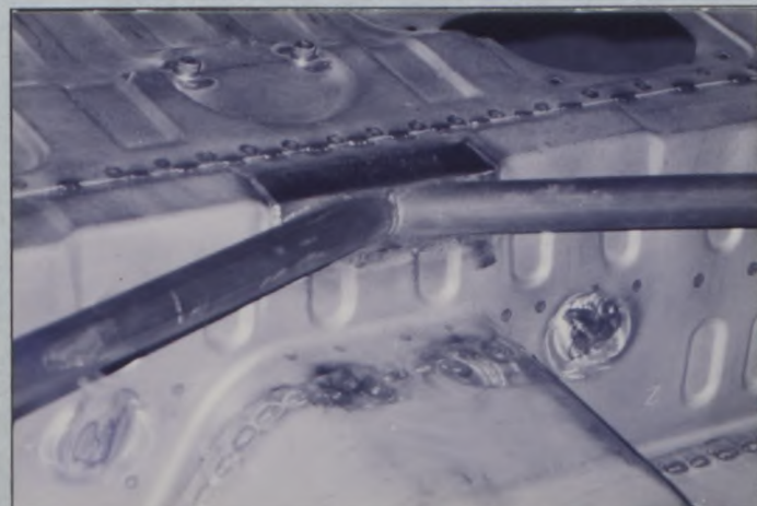
PHOTO No. 7 Central framework to floor
