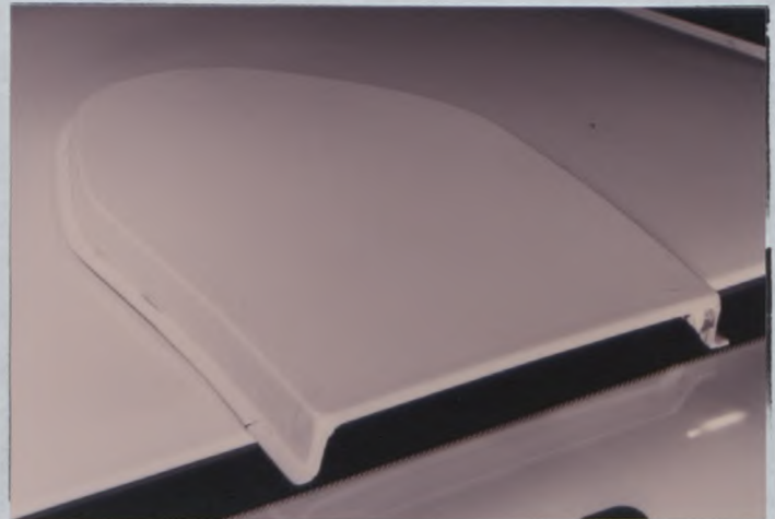
PHOTO No. 8 ROOF VENTILATION
