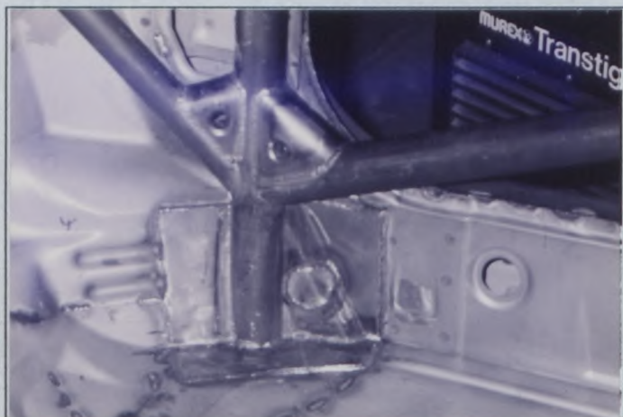
PHOTO No. 7 Lateral bar to floor
