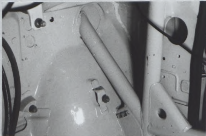
Front reinforcement to bulkhead
