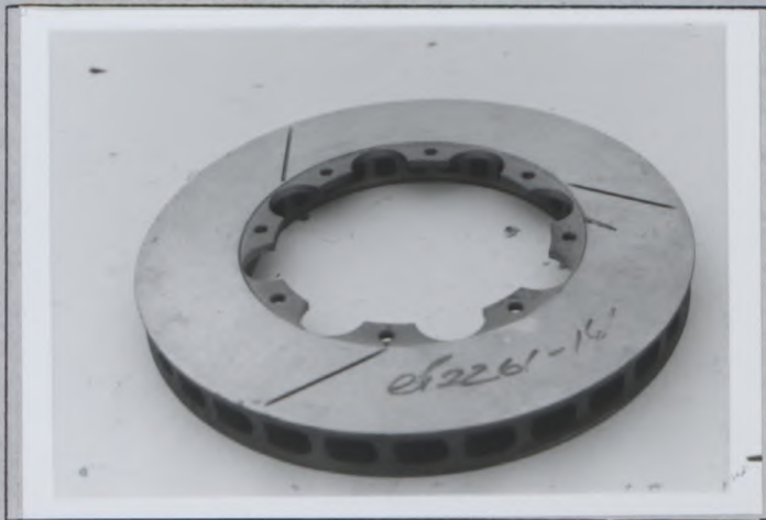
Photo V2 Front brake disc
