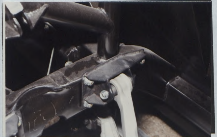
PHOTO No RIGHT MAIN ROLLBAR WELDED TO FRAME
