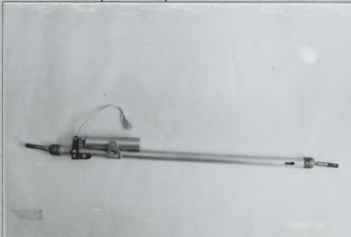
Z3 Elec, power cylinder for rear
