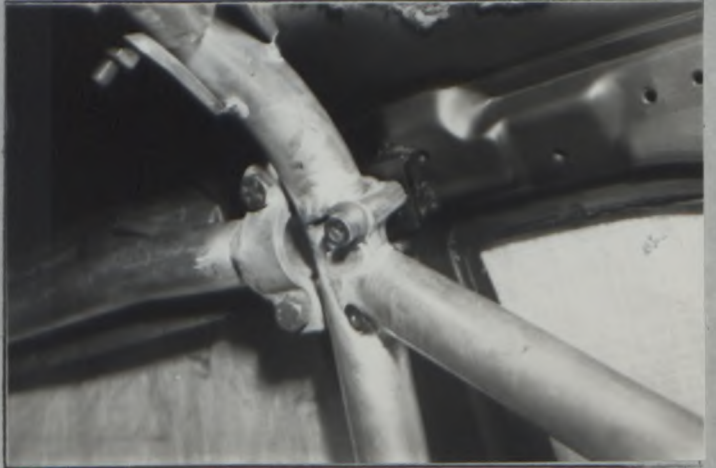
Main hoop to roof
