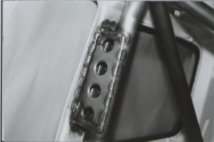
PHOTO N° 6 Main hoop to pillar
