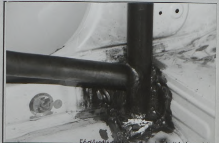
PHOTO N° 5 Main hoop to floor
