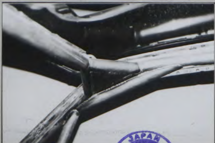
PHOTO N° 10 FRONT LATERAL TO ROOF (RIGHT)
