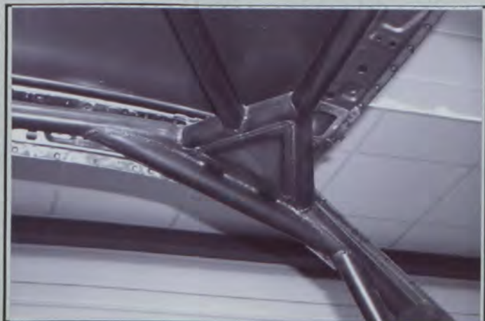
PHOTO N° 8 FRONT LATERAL TO ROOF (LEFT)
