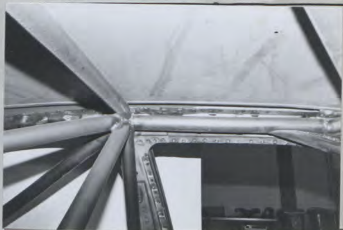
PHOTO N° 7 MAIN HOOP TO ROOF (LEFT)
