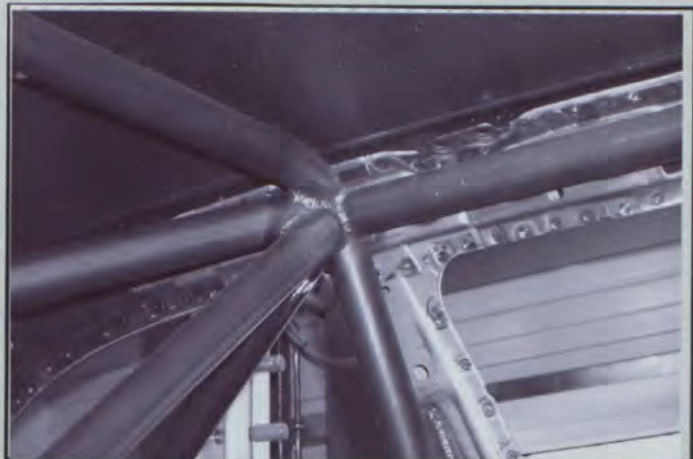
PHOTO N° 6 MAIN HOOP TO ROOF (LEFT)
