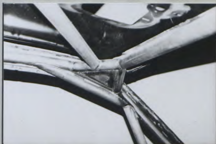
PHOTO N° 9 FRONT LATERAL TO ROOF (LEFT)
