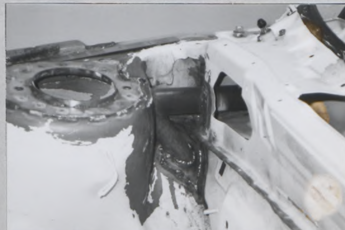
PHOTO No.10 Front framework to turret
