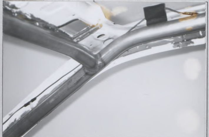
PHOTO No. 2 Lateral bar to A-pillar
