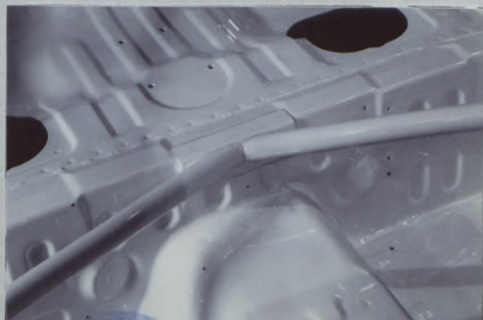
PHOTO N° 5 CENTRAL FRAMEWORK TO FLOOR
