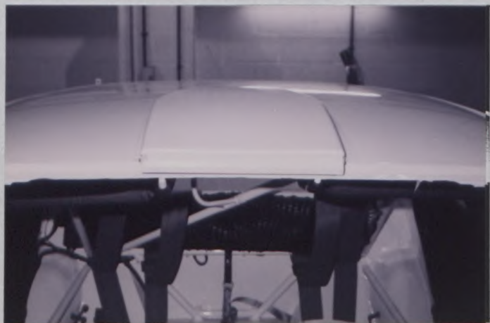
PHOTO No. 117 FLAPS FOR VENTILATION
