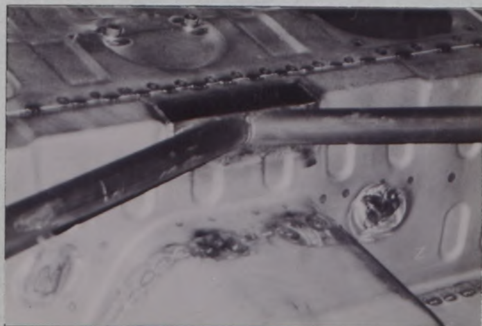
PHOTO No. 5 Central framework to floor
