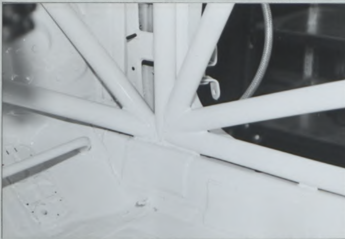
PHOTO No. 7 (FRONT HOOP TO FLOOR)
