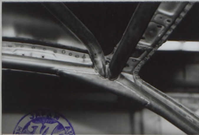
PHOTO No. 7 (FRONT LATERAL TO ROOF)
