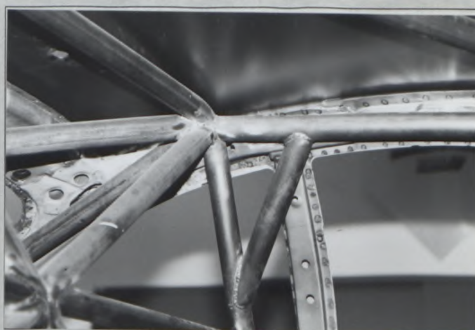
PHOTO No. 4 (MAIN HOOP TO ROOF)
