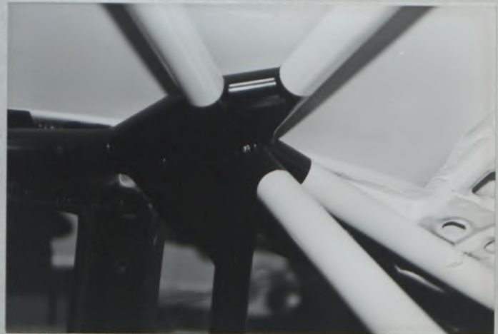
PHOTO No. 4 (MAIN HOOP TO ROOF)
