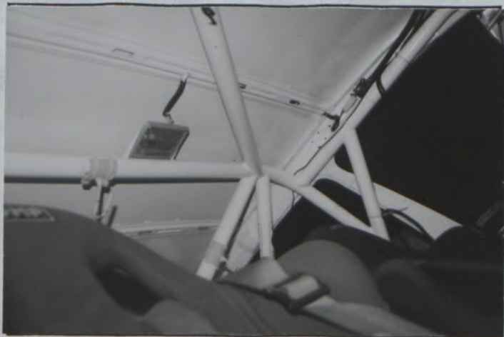
PHOTO No 5 Main/Lateral/Diagonal bar joint
