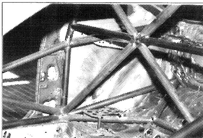
PHOTO No. 14 (REAR FLOOR SECTION)
