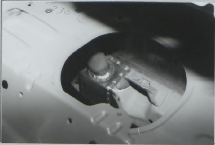
PHOTO No 15 Rear support bar to Rear floor
