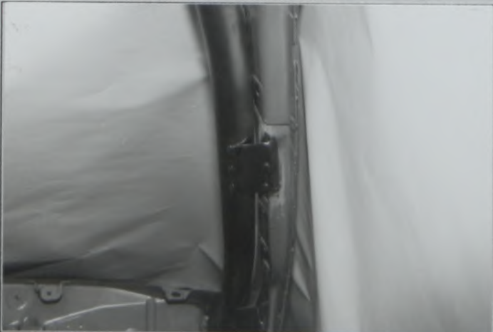
PHOTO No 5 Front hoop to Front pillar
