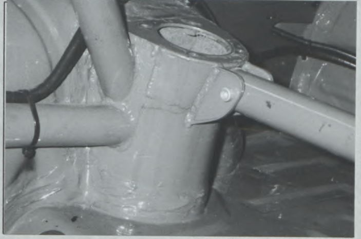
PHOTO H) REAR SUPPORT TO TURRET
