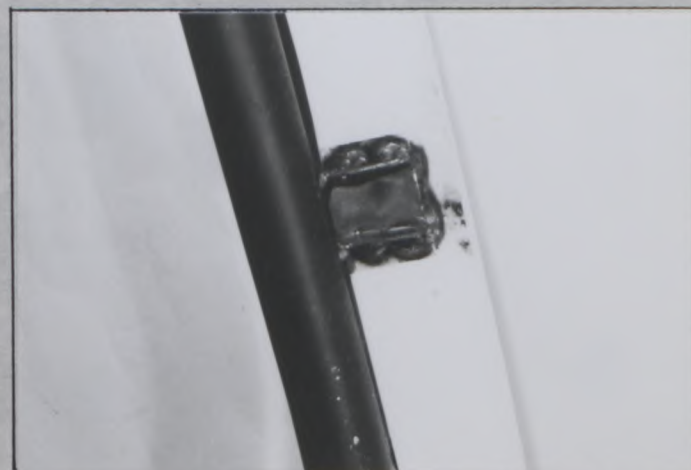
Main hoop to pillar
