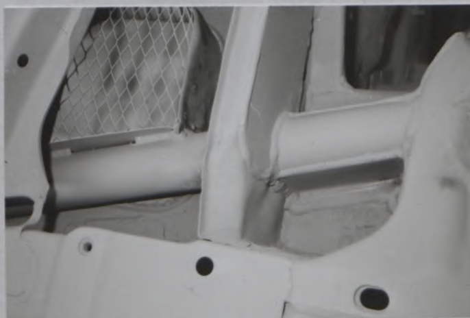
Front reinforcement to front strut tower
