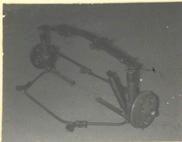
Front axle complete (without wheels).
