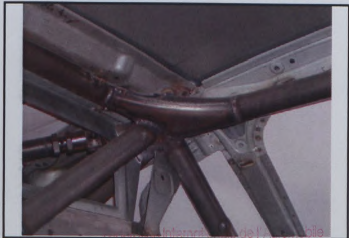
PHOTO N° 11 main roll bar to longitudinal member and rear diagonal removable member (left side)
