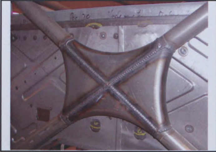
PHOTO N° 12 cross diagonal members
