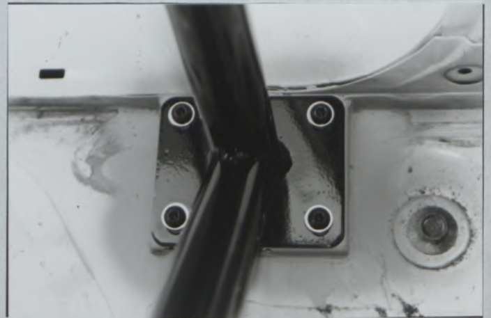
PHOTO N° 3. Main hoop to floor LH
