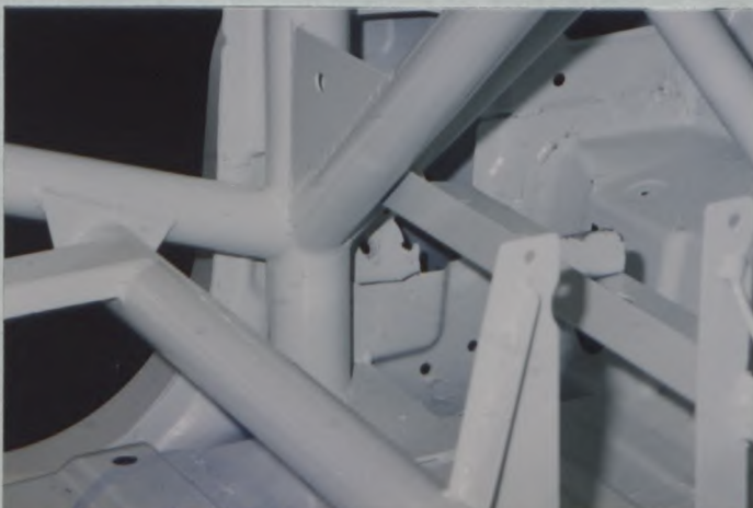
PHOTO N° 4 MAIN HOOP TO FLOOR-RIGHT
