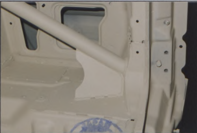
PHOTO N° 10 REAR SUPPORT BAR TO FLOOR
