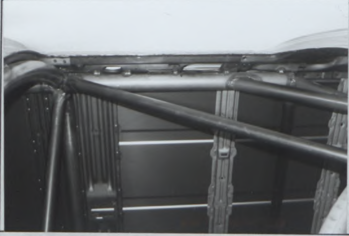
PHOTO No. 13 Rear hoop to roof side
