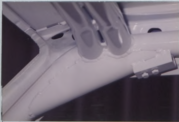
PHOTO No. 8 FRONT HOOP TO ROOF
