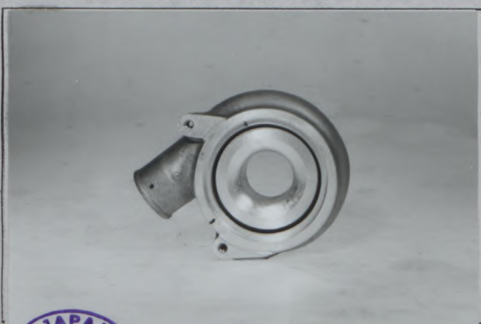
Q) Impeller housing of turbocharger
