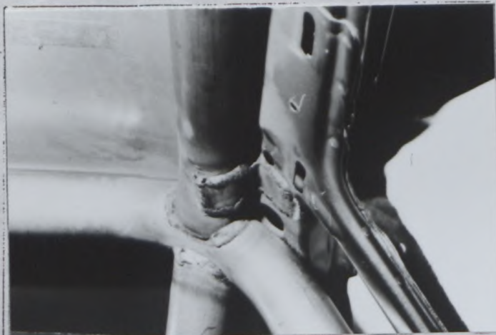
Main hoop to roof
