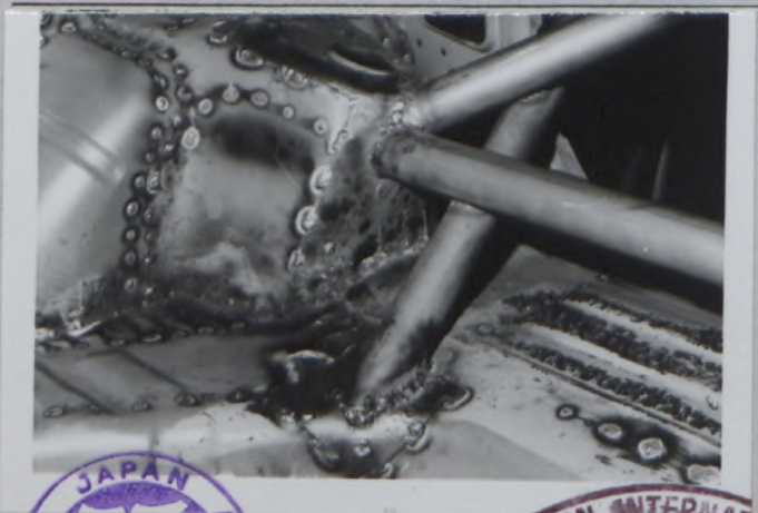
Rear left hand support to floor, and rear diagonal rollbar and rear lateral rollbar to shock absorber tower
