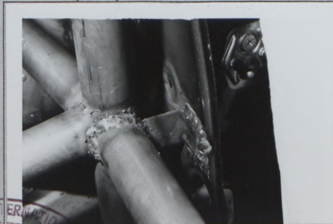
Main hoop to pillar
